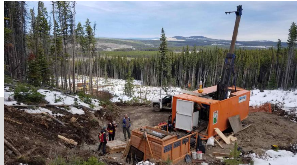
Highland Valley Drilling, fall 2020
